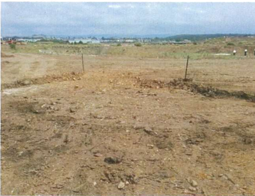
Photograph 6: Ground surfaces in the location of Area P3 following removal of asbestos stockpiles to the containment cell.
