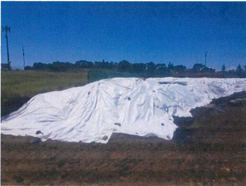
Photograph 2: Geofabric encapsulation over ACM impacted soils within containmant cell.
