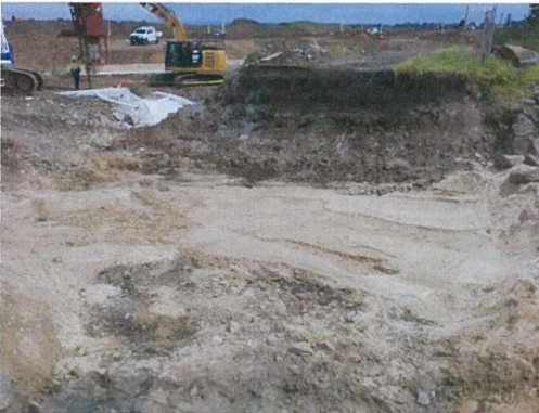
Photograph 5: Ground surfaces in the location of former bridge following removal works.
