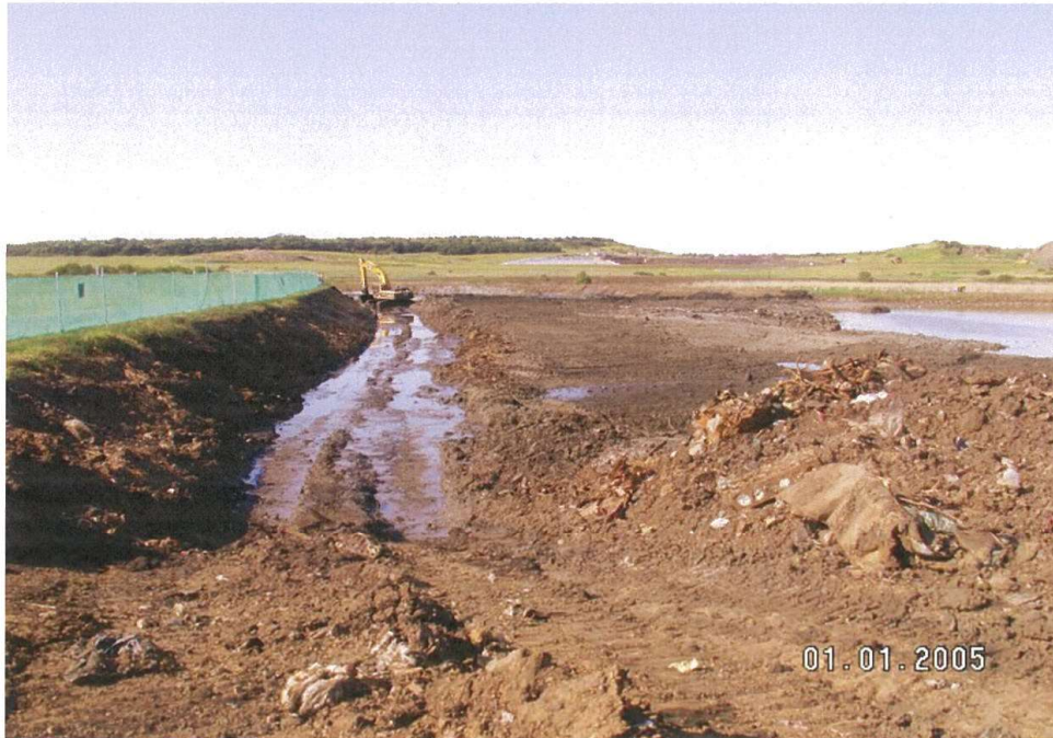
Photograph of the audit Site adjacent to Keith Hockey Field which is near the recent un-expected find area taken 4/10/2017 (note date stamp on photo is incorrect)
